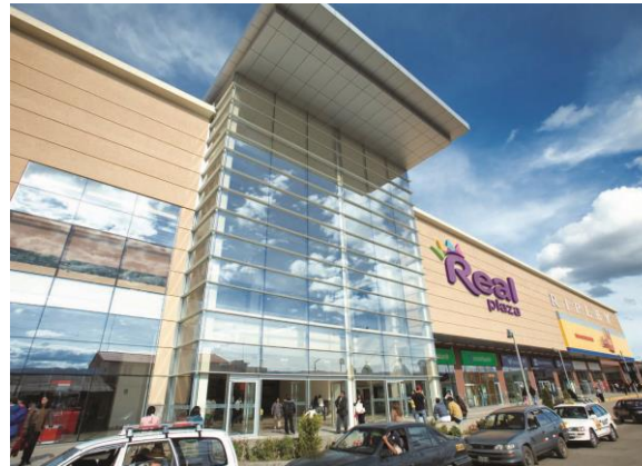
Expansions of existing malls
